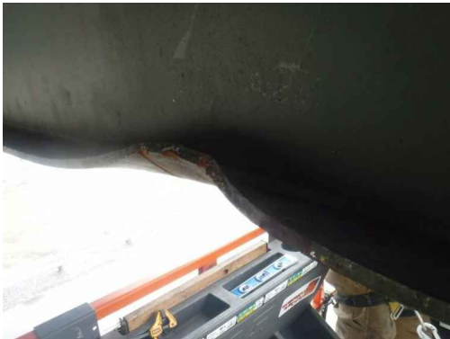
PHOTO - P5 BEAM 5 - BOTTOM FLANGE DAMAGE
