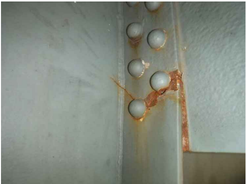
PHOTO - P4 BEAM 1 - CRACK IN CONNECTION P
