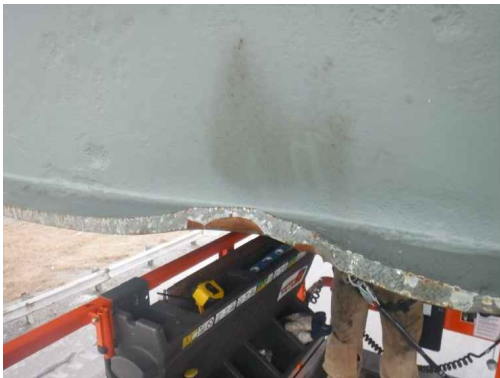
PHOTO - P7 BEAM 4 - BOTTOM FLANGE DAMAGE
