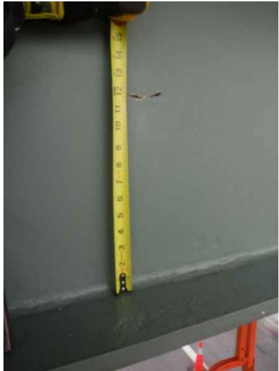
PHOTO - P2 BEAM 1 - HORIZONTAL CRACK IN WEB
