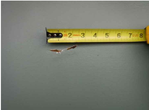
PHOTO - P3 BEAM 1 - HORIZONTAL CRACK IN WEB
