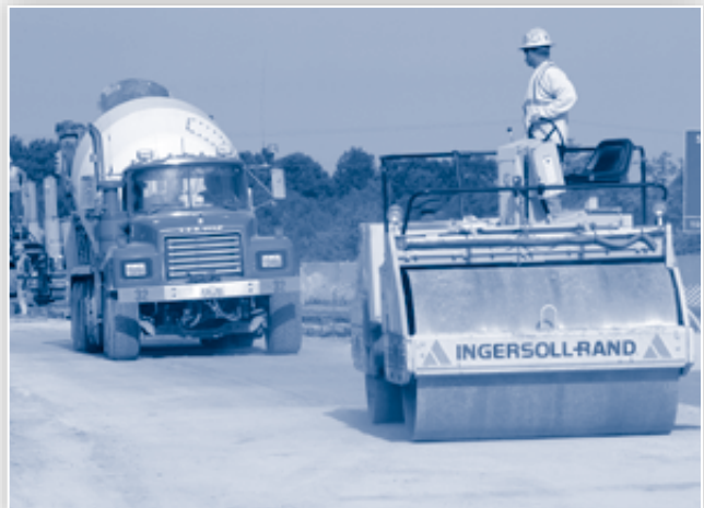
Ongoing construction for the State Route 58 Interchange (#140).
