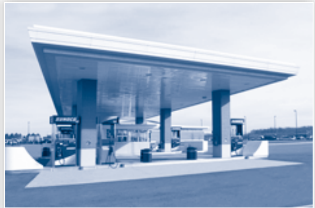
New fuel islands at the reconstructed plazas offer service to multiple customers.
