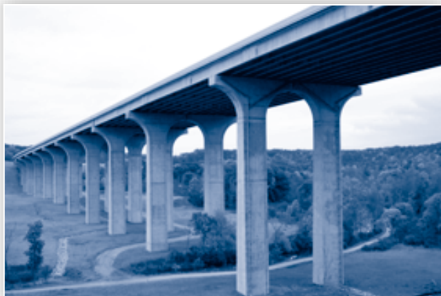
The Cuyahoga River Bridges span 2,682 feet above the Cuyahoga Valley National Park in Summit County.
