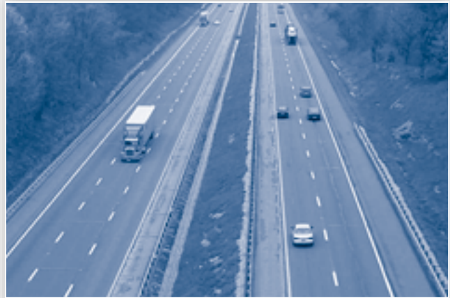
This portion of the Turnpike roadway shows a new third-lane section and a two-lane section which has yet to undergo construction.
