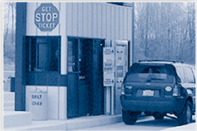
At the renovated toll plazas, travelers receive their toll ticket from a dual automatic ticket-issuing machine.
