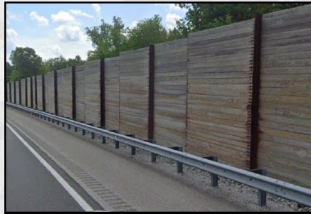
BRECKSVILLE NOISE BARRIER
