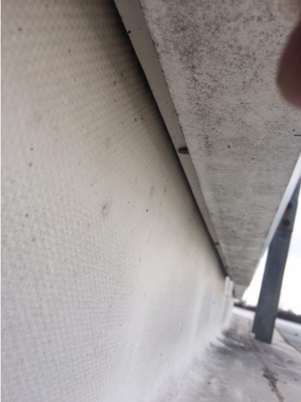
Bottom of Fiberglass Fascia w/exposed fasteners:
