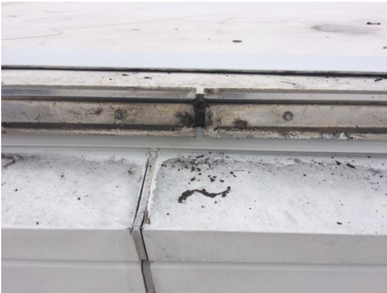
Top of Fiberglass Fascia w/metal trim removed:
