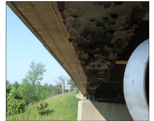
PHOTO 1 - LOOKING WEST AT BEAM 5
