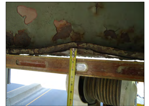
PHOTO 2 - LOOKING SOUTH AT BEAM 4
