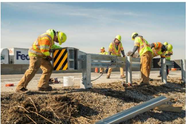
End Terminal Assembly Replacement
