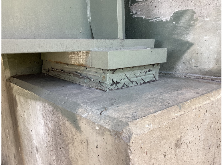
Typical OTIC Elastomeric Bearing
