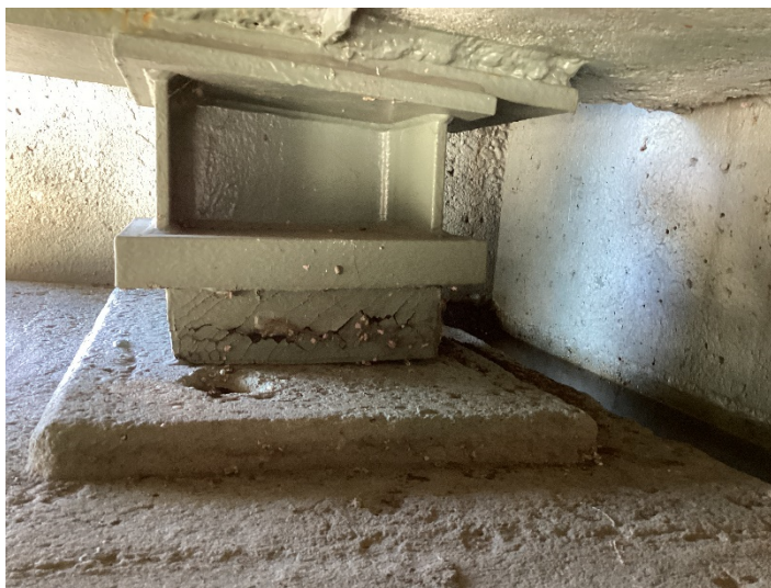
OTIC Bearing Replaced with Elastomeric Type
