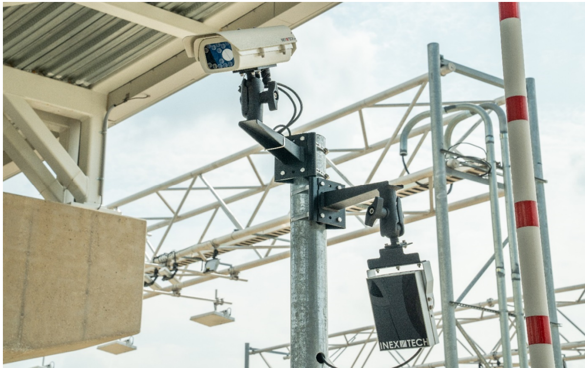
Cameras at Electronic Tolling Gantry
