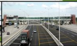
Cash, Credit, E-ZPass & Open Road Tolling
